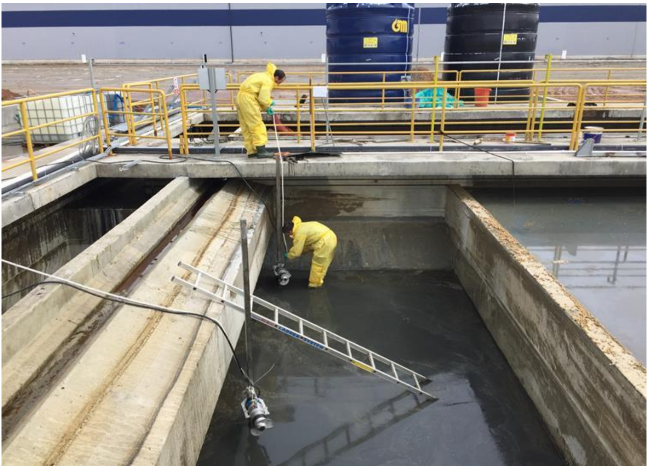
Settling Basin Mixers and Oil Stripping Construction
