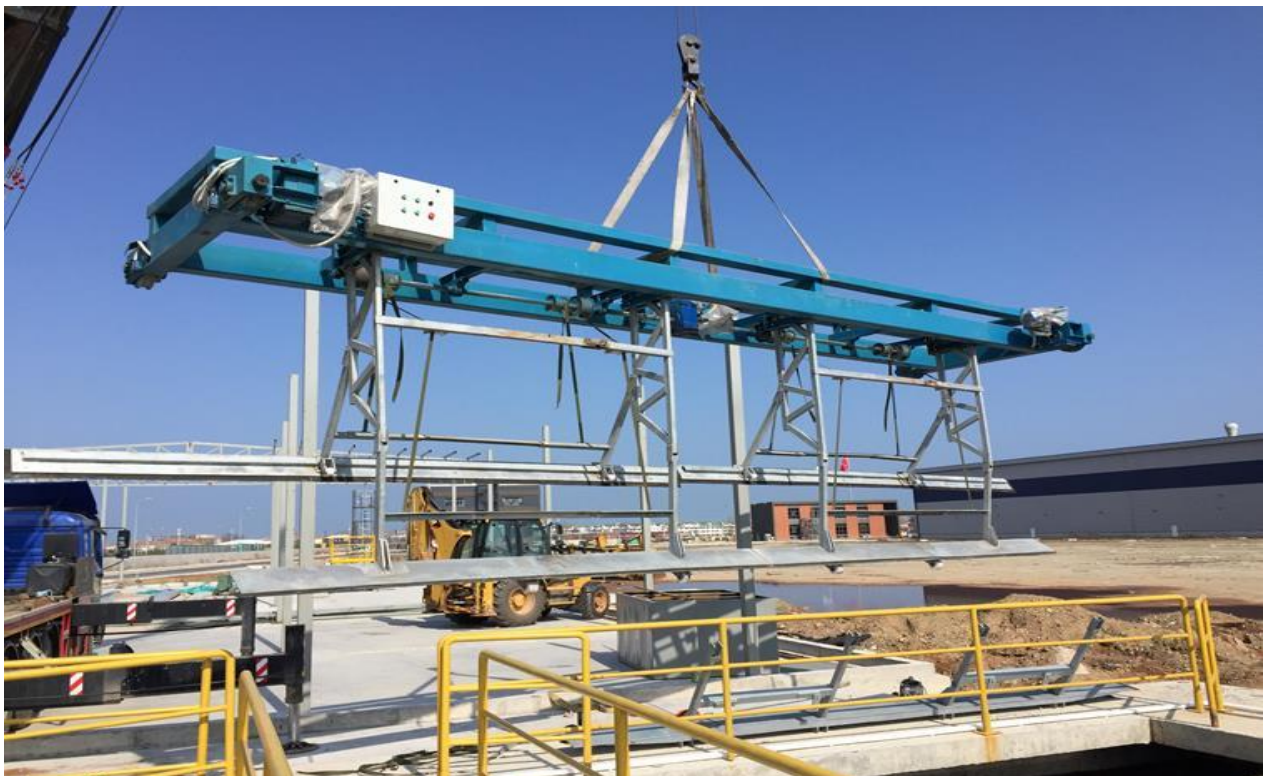
Settling Basin Scrapper Bridges Installation
