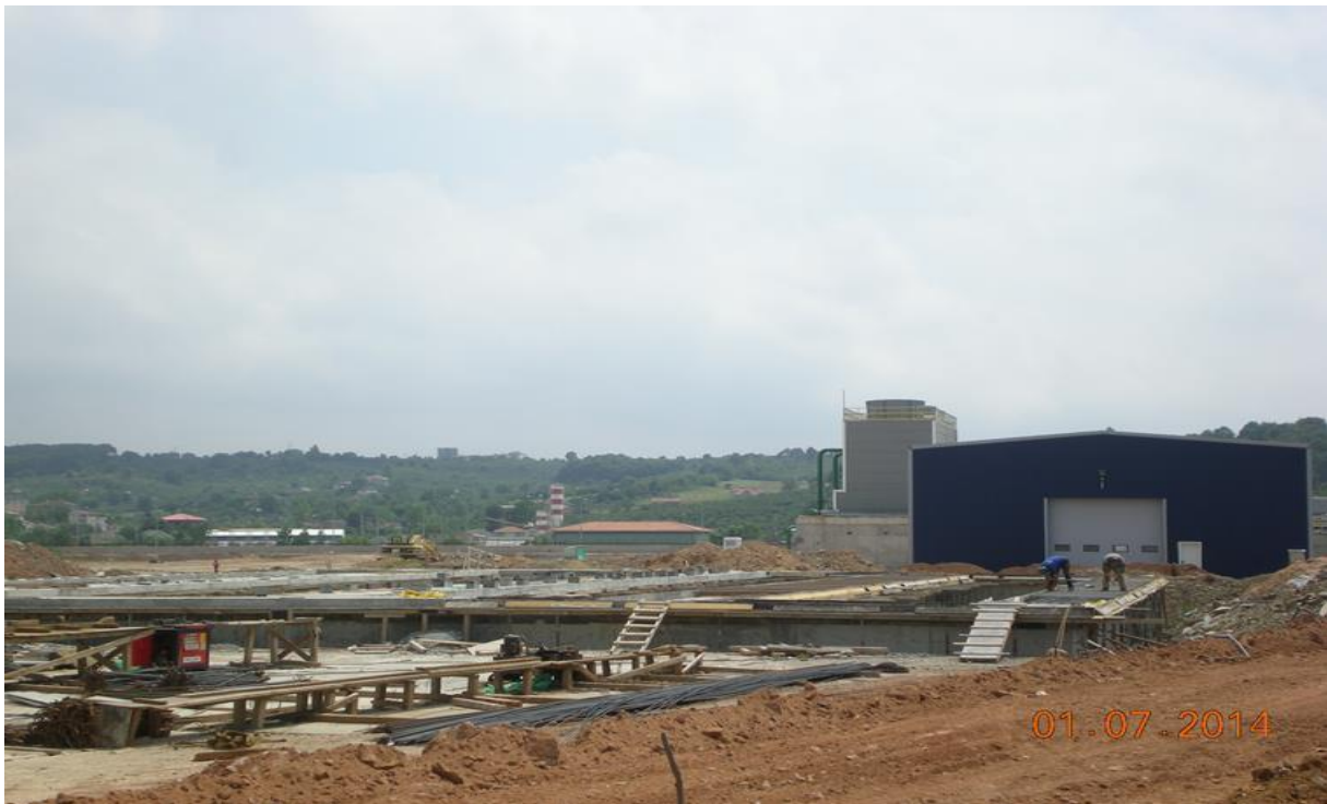
Water Treatment Plant and Chemical Treatment Plant General Appearance
