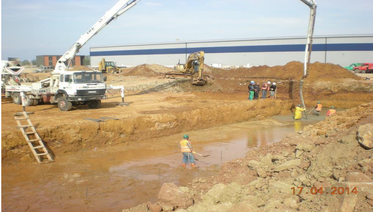
Chemical Treatment Plant Excavation and Grobeton Pouring
