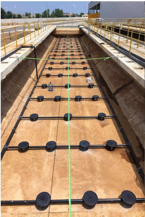
Blowers Air Bubbles - Microbiological Treatment Basins
