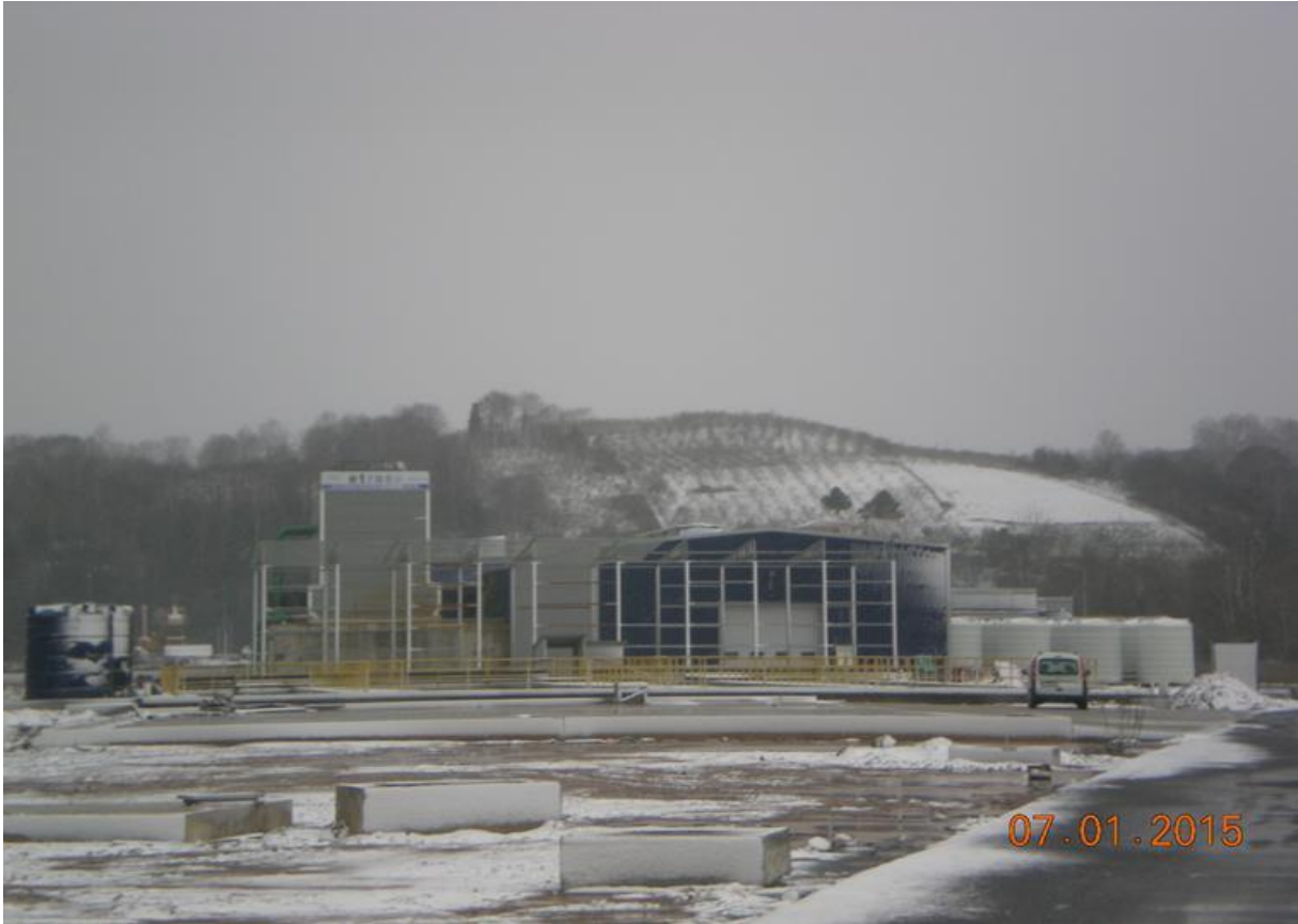
Water Treatment Plant and Chemical Treatment Plant General Appearance
