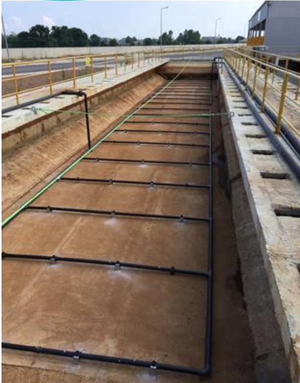
Chemical Treatment Plant - Microbiological Treatment Basins
