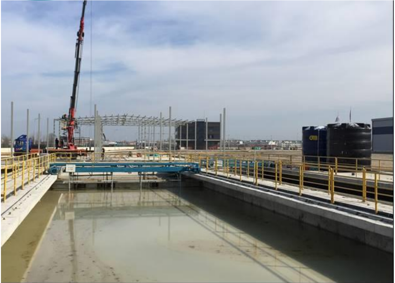
Settling Basin Scrapper Bridges Instalation
