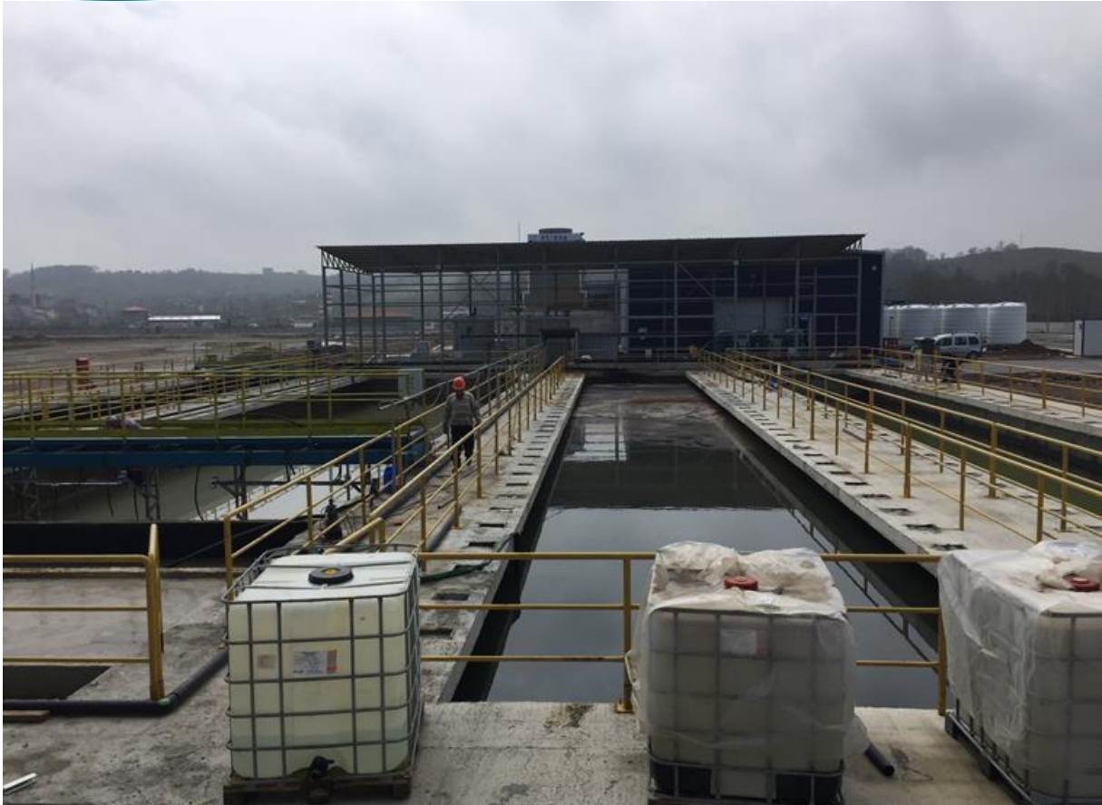
Water Treatment Plant and Chemical Treatment Plant General Appearance
