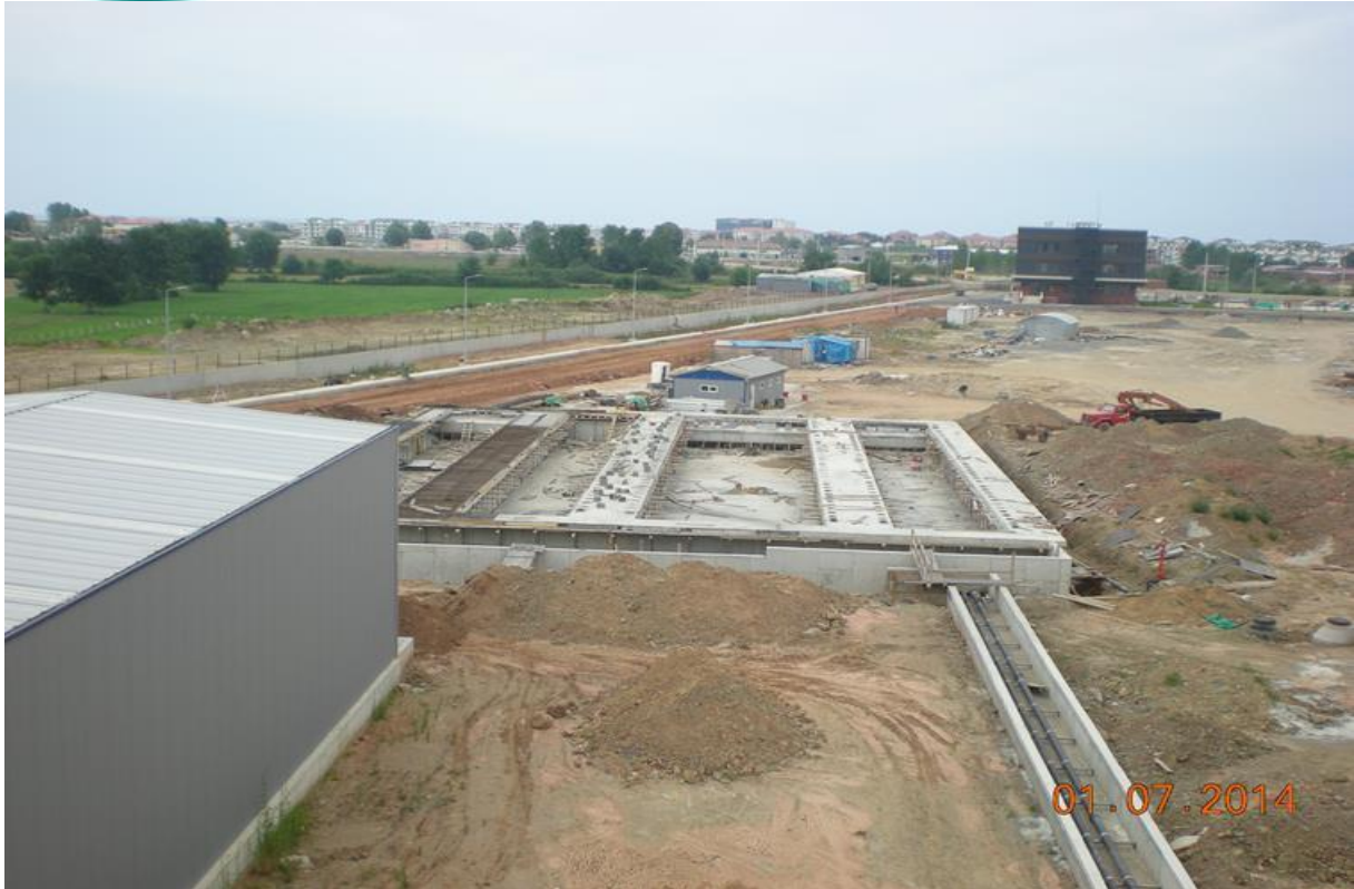
Water Treatment Plant and Chemical Treatment Plant General Appearance
